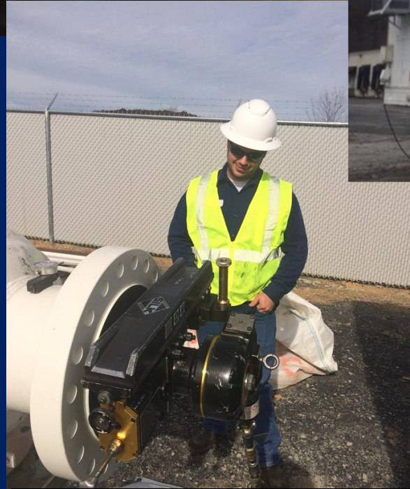
On Site Flange Resurfacing
