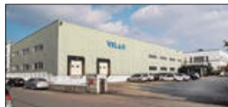
Ansan City, South Korea Velan Ltd., Plant 2
