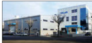
Ansan City, South Korea Velan Ltd., Plant 1
