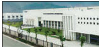
Suzhou, China Velan Valve (Suzhou) Co., Ltd.
