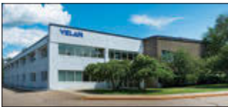
Williston, VT, U.S.A. Velan Valve Corp., Plant 3
