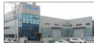
Ansan City, South Korea Velan Ltd., Plant 3
