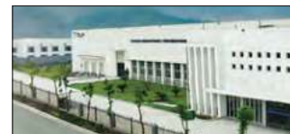
Suzhou, China Velan Valve (Suzhou) Co., Ltd.
