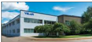
Williston, VT, U.S.A. Velan Valve Corp., Plant 3
