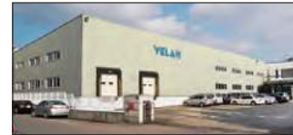
Ansan City, South Korea Velan Ltd., Plant 2
