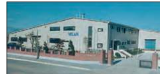
Ansan City, South Korea Velan Ltd., Plant 1
