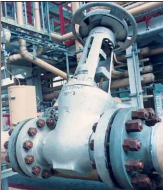
Pressure seal valves used in oil and gas applications.
