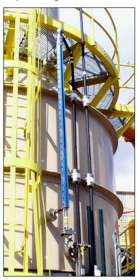
Specifically designed for low pressure, light duty applications, the new Jerguson Mini-Magnicator is a great replacement for fragile tubular glass. The Mini-Magnicator provides the same easy to read level indication as the Jerguson Magnicator, in a smaller more economical package. The Mini-Magnicator utilizes the standard Jerguson latching flag design –
